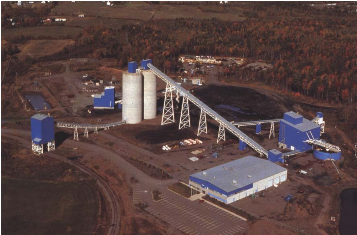
Figure 2 Aerial view (pre-explosion) of Westray mine site (from Richard, 1997).
